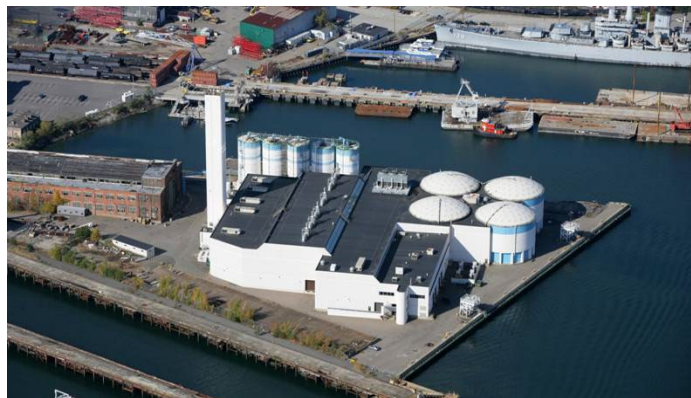
Figure 1: MWRA's Pelletizing Plant
